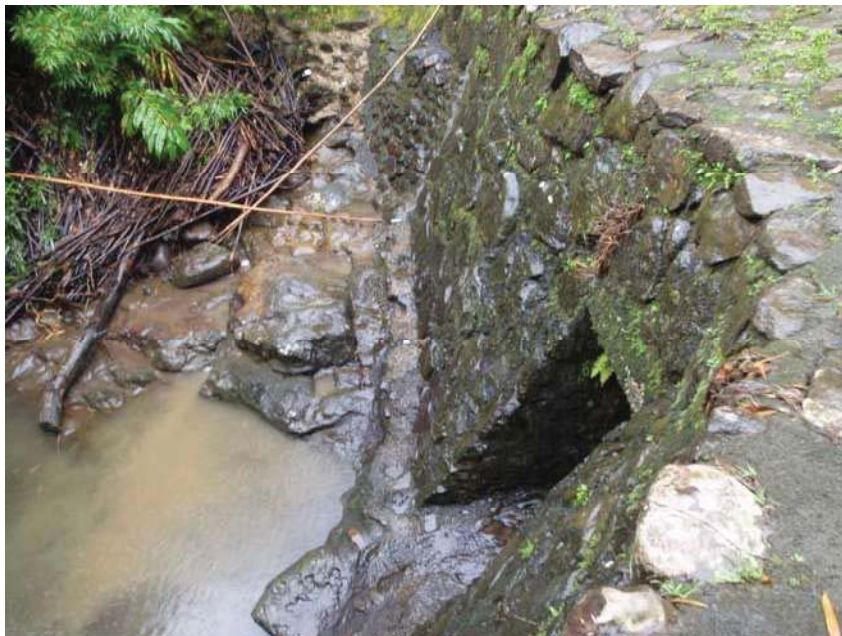
Figure 4-7. Photo shows below the diversion and is taken across the stream. Note there is only a trickle flowing from the gate. (3/12/2009; Tributary name: Kōlea (64003001); PBN: dk003p-017-031209; Surveyor: Kuamo‘o, D.; SBN: dk003n-031209; Lat. (DD): 20.87282, Long. (DD): -156.19005).
